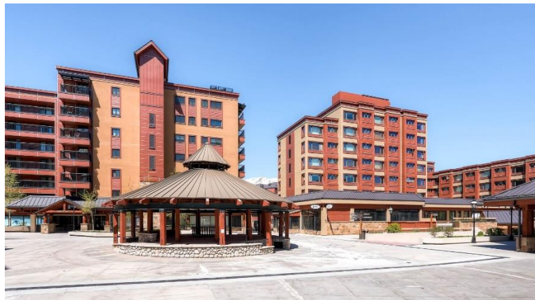
Figure 4. The surrounding modernist buildings only serve to further highlight the regionalist style of the fire pit.
