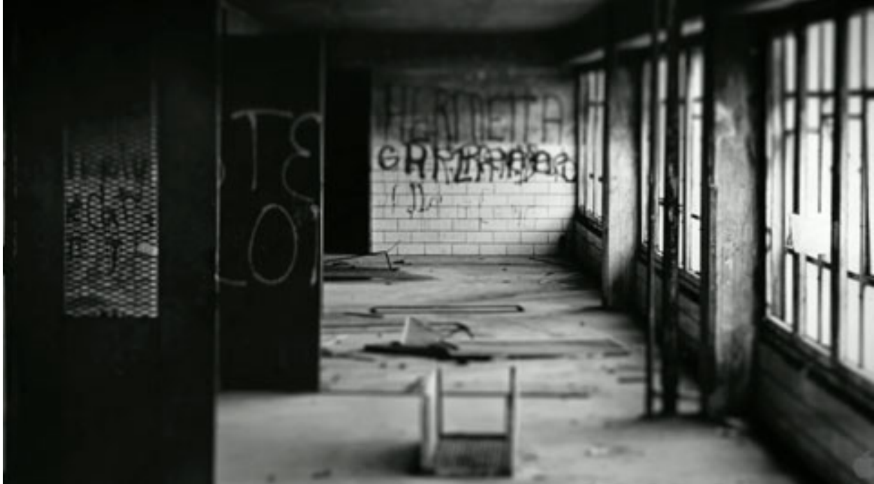
Figure 4: An interior hallway at Pruitt-Igoe, courtesy of Pruitt Igo Now.
